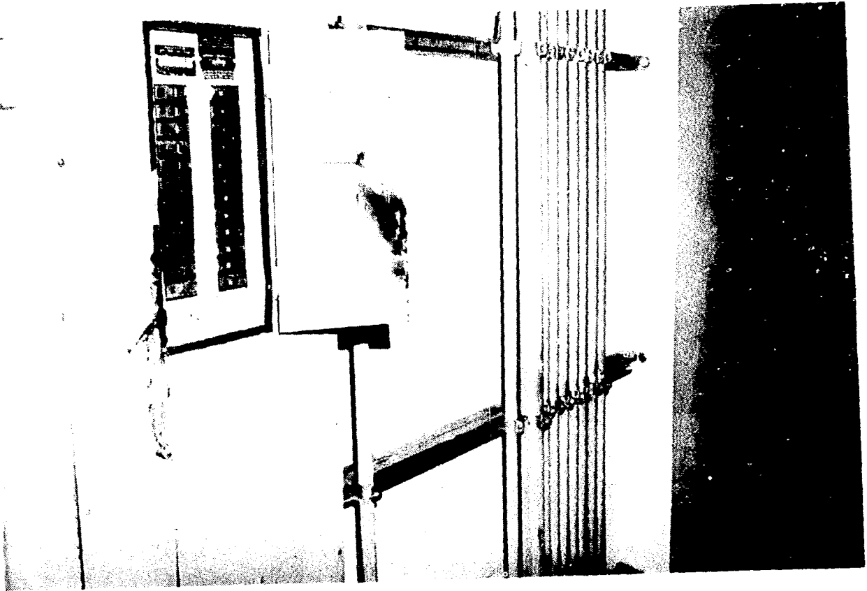
Figure 22. Charring and melted door seal material on electrical panel in southeast area of the 347-foot elevation.
