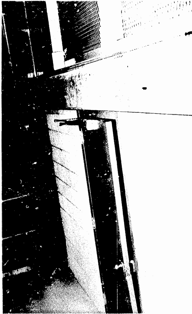
Figure 5. Door on 325-foot elevation with broken latch; door forced open by overpressure.
