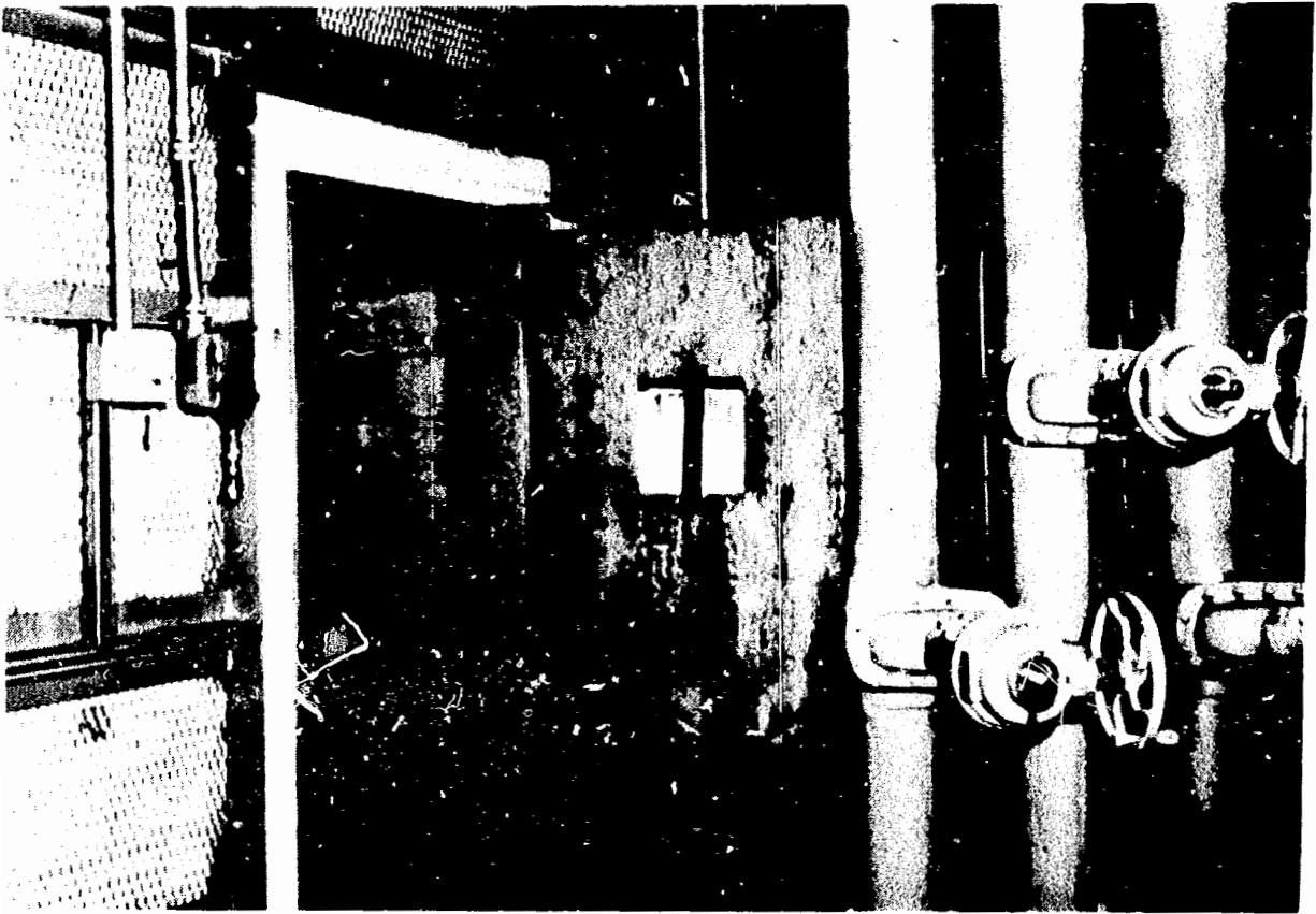
Figure 3. Enclosed stairwell door on the 305-foot elevation indicating overpressure damage.
